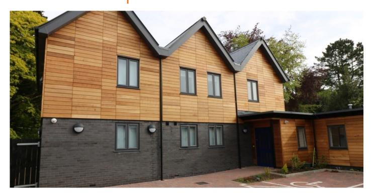
Demolition of annex building; construction of new two storey block with a single storey link to the main house. New Construction to be pitched or flat roofs with masonry cavity walls with a combination of facing brick and timber cladding to elevations; timber upper floor and roof structure; Double glazed uPVC Windows; plastered wall & ceiling finishes internally.
