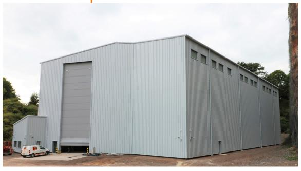
The construction of specialist warehouse facility, consisting of a steel framed measuring hall clad with plastic coated cladding sheets, secured down to the existing rock with large concrete pad stones. The structural floor inside is constructed of concrete with steel reinforcing, with a turntable and tracking pit incorporated into this. The ground floor slab level required specialist precision works to ensure tolerances of less than two millimetres across the 38m by 52m floor space.
