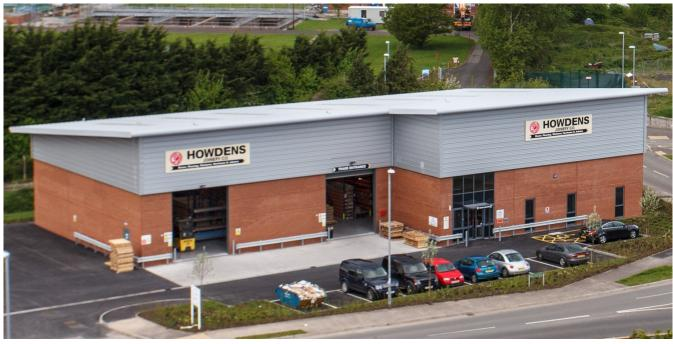
The works comprised ground improvement to area of proposed building, enabling pads and trench fill foundations to be constructed. Superstructure comprises steel frame system with blockwork infill panels and external brickwork to 4.8m in height. The building clad with composite preformed insulated metal panelling and roof coverings with 10% area of roof light. Floor slab comprised reinforced concrete with power float finish and sealant and design loading of 30KN/m2.
