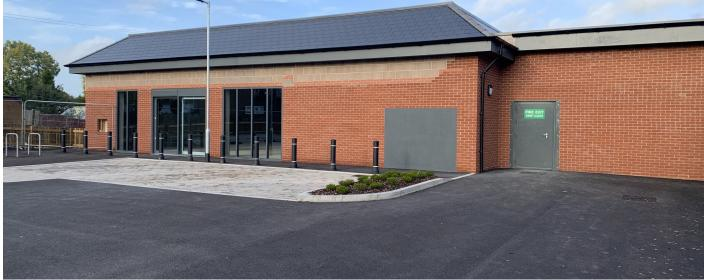
A New Single storey food retail unit approx. size 400m2, consisting of steel frame on strip foundations with a suspended precast concrete floor slab, Brick / Block external walls and pitched tiled roof to the retail space and flat Roof to the stock chiller room area. External glazing and doors.
