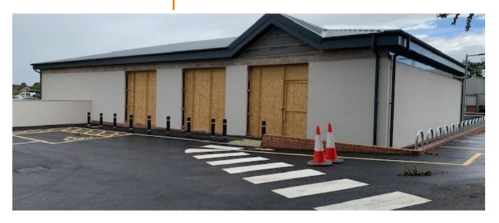
The works involved the erection of a new store shell and associated car parking. The store consists traditional concrete foundations with Masonry cavity fair faced blockwork and brickwork part rendered externally. The internal blockwork has been painted to RAL 7043. The ground floor slab is Concrete pre-cast slab units with insulation and screed over.
